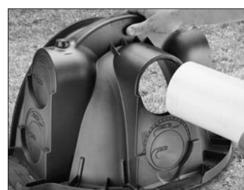
5. Insert inlet pipe.
