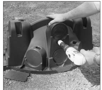
2. Drill hole with hole saw.
